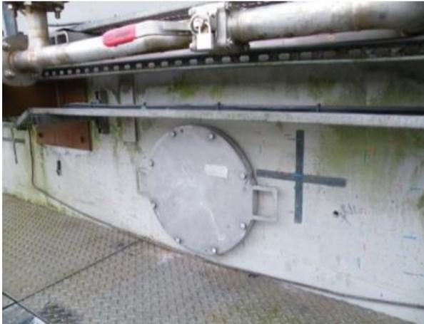
Fig. 4. One of the penetrations in the FSTR, representing the new penetrations in the North & South walls.
